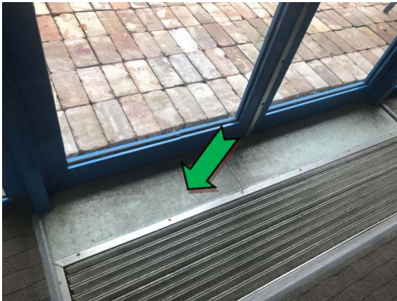
Photo 9. Interior, ground level, playroom, blue floor coverings – suspected non asbestos-containing sheet vinyl.
