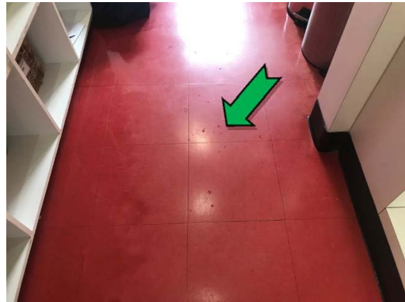
Photo 10. Interior, ground level, change room, red floor coverings – non asbestos-containing floor tiles.
