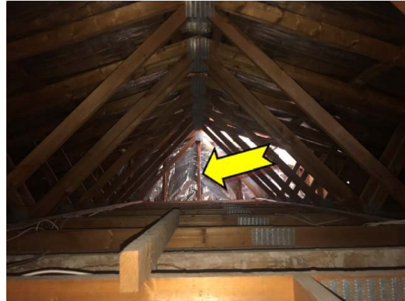
Photo 14. Interior, level 1, roof space, gable end – suspected SMF sarking insulation.
