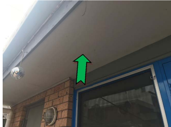
Photo 2. Exterior, ground level, north elevation, eaves – non asbestos-containing fibre cement sheeting.
