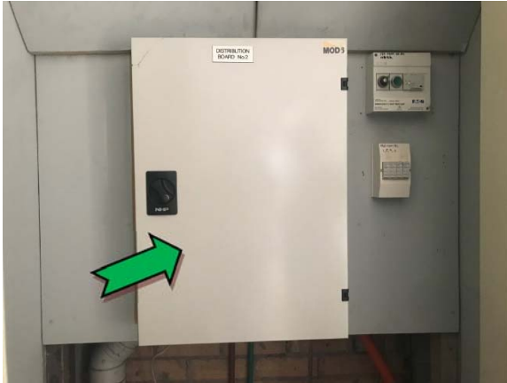
Photo 7. Interior, ground level, electrical cupboard – suspected non asbestos-containing bituminous backing board.
