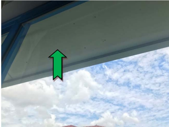
Photo 1. Exterior, level 1, north elevation, eaves – non asbestos-containing fibre cement sheeting.
