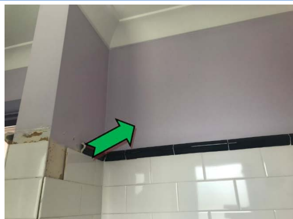
Photo 6. Interior, level 1, bathroom, walls – assumed non asbestos-containing fibre cement sheeting.
