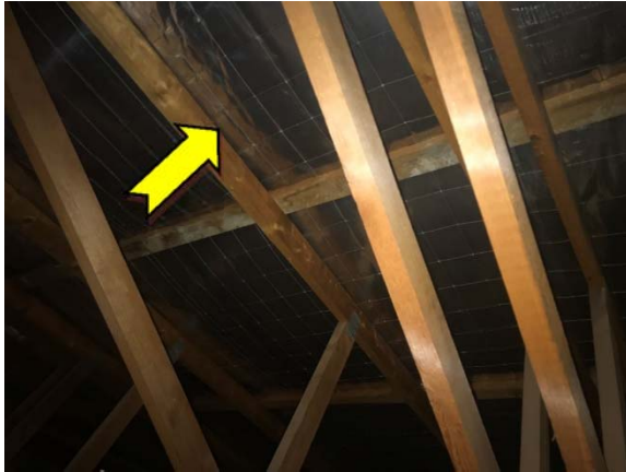
Photo 13. Interior, level 1, roof space – suspected SMF sarking insulation.
