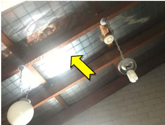
Photo 15. Interior, ground level, storeroom, ceiling space – suspected SMF sarking insulation
