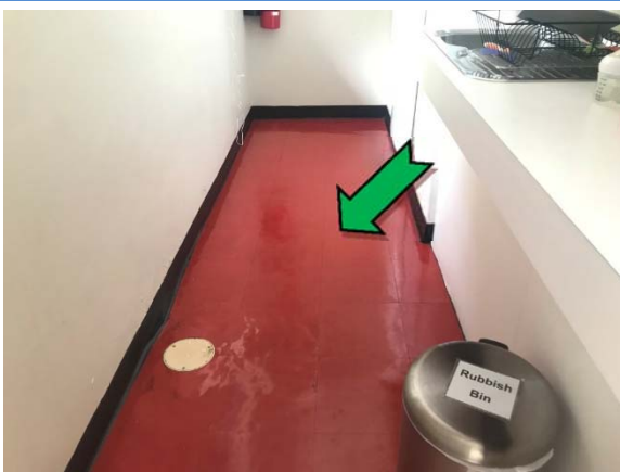
Photo 11. Interior, ground level, office, red floor coverings – assumed non asbestos-containing floor tiles.
