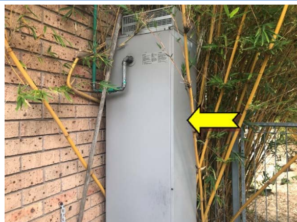
Photo 12. Exterior, south-west elevation, hot water heater – suspected SMF internal insulation.
